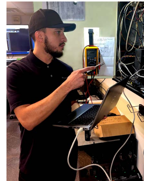
Nick Sanchez, a 2022 graduate of the Building Automation Systems training program was hired by Climatec within a week of completing the program.
